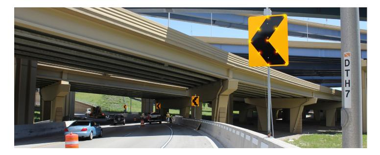
Due to the proven success of the curve warning system at that location, WisDOT installed the system with sequentially flashing signs at another one of the busiest interchanges in the state, the Zoo Interchange, when it was being completed in fall 2017. Since then, the interchange has experienced fewer collisions than the statewide average, despite the high traffic volume.
